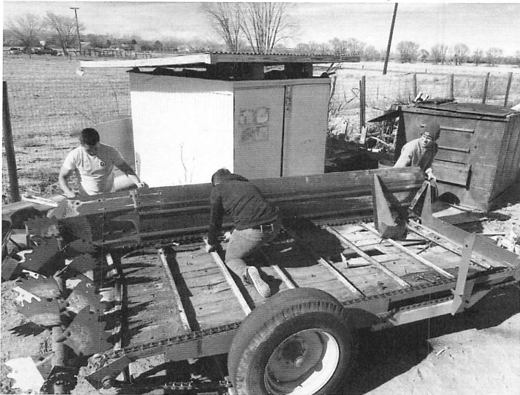
Figure 1: The trailer being converted to support solar panels for future on-the-go charging of equipment. One of the student groups worked on this community project.
